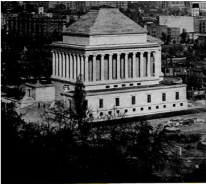
View of Building, Showing Solid Limestone Roof
